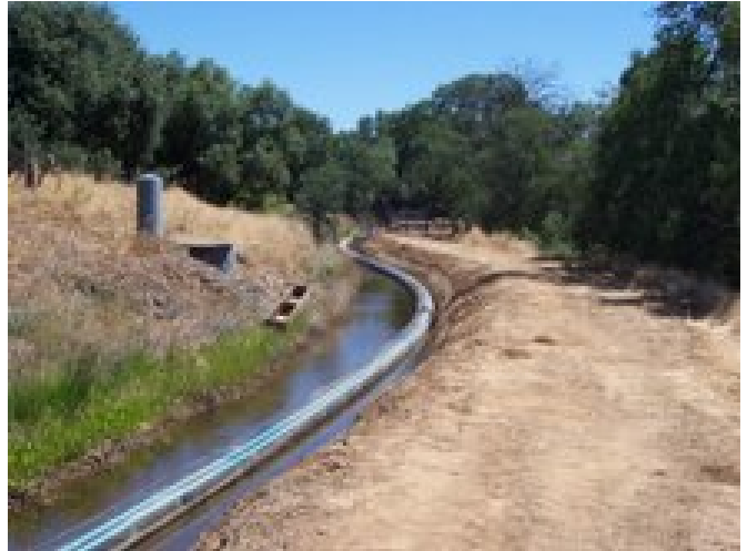
The treated waterline seeks to replace an open raw conveyance to 109 households.
