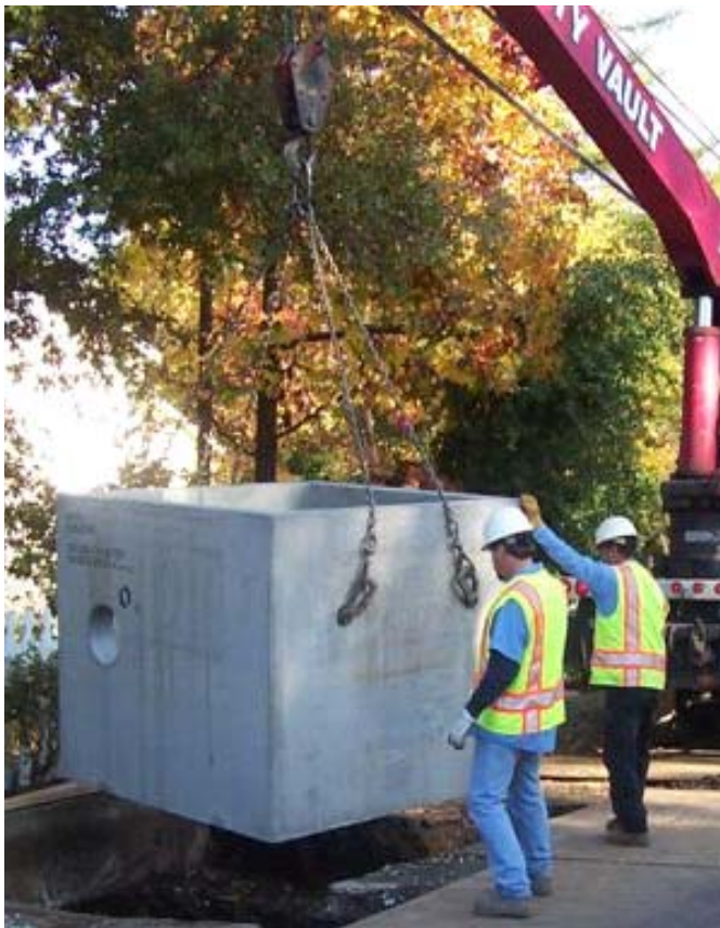
The vault weighs 8,400 lbs. The lid for the vault is equipped with springs and hydraulic lift assistance making it nearly self opening after safety devices are turned to allow the cover to open.
