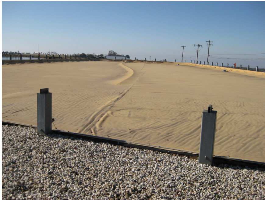
Figure 1: The existing geomembrane floating cover on the 2-million gallon Tanner finished water storage reservoir will be replaced in spring 2010 with a new floating cover that will continue to protect the quality of water in the reservoir. Note: The curve in the center of the cover is an underwater floating baffle. It improves water circulation through the reservoir.
