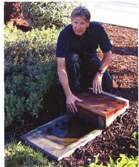
AWA's Barry Birge shows off the features of the wildlife hydration station he designed with suggestions from Joe Aparicio. The concrete basin is shallow at one end for birds and small animals, and deeper at the other end for deer and larger animals. A wooden cover protects the float and valves, and offers shade for small fish. The sample hydration station is installed in the Demonstration Garden at the Water Agency office.
